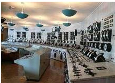
Figure 2 a Pre-DCS/SCADA Era Central Control Room
